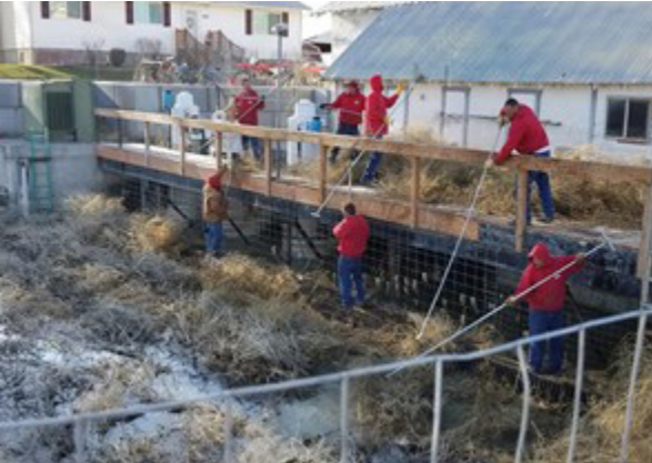
A large crew manually removes tumbleweeds from the original screening system in the Owsley canal.
