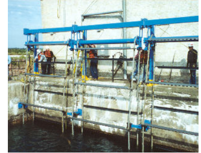
I-Beam mounting for Rake Only model
