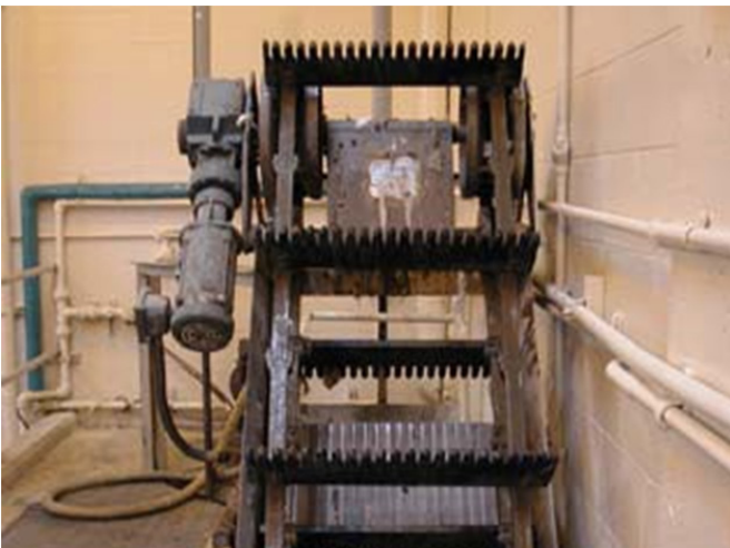
The Duperon ® FlexRake ® FP was commissioned in 1998 and has been running strong, and maintenance-free for over 20 years.
